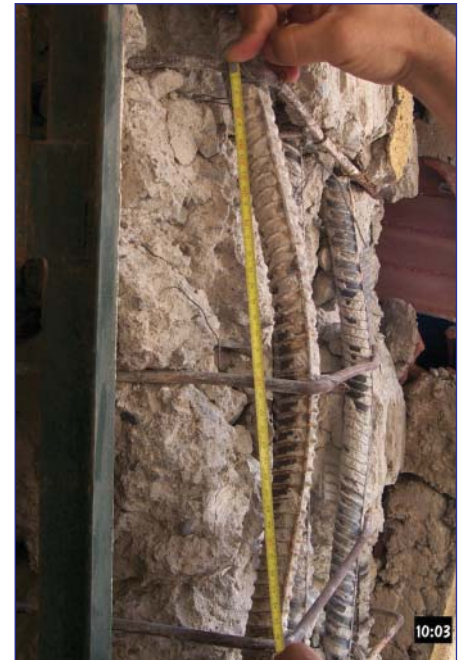
Figure 5: Non adequate detailing
