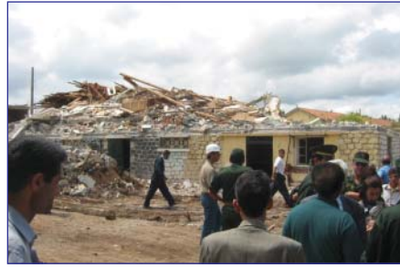
Figure 3: Non tied stone masonry
