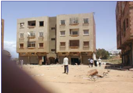
Figure 2: Soft (first) storey
