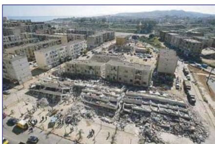
Figure 2: Building damages observed in the city of Boumerdes
